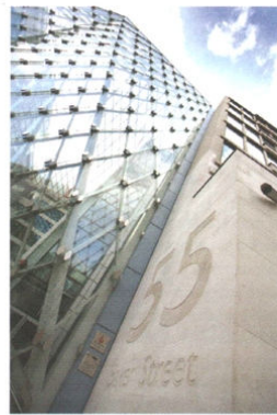
The former Marks & Spencer HQ uses Aermec free-cooling chillers
